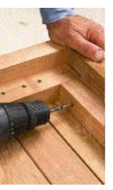
faces of the end 2-by-4s with three 21/2-inch screws. Measure width and length between the end and side ledgers, then subtract 1/4 inch from each for dimensions of base. Cut frame sides and ends from ripped-down 2-by-6s.
