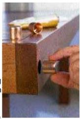
sides and into tabletop side ledgers. Epoxy copper caps in exposed holes.
