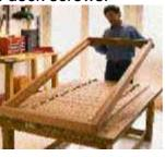
by-3s with cardboard spacers still in place. It should be a tight fit. Add a pair of spacers between frame and first board at each end. 4. Butt 2-by-4 side pieces over 2by-4 end pieces.
